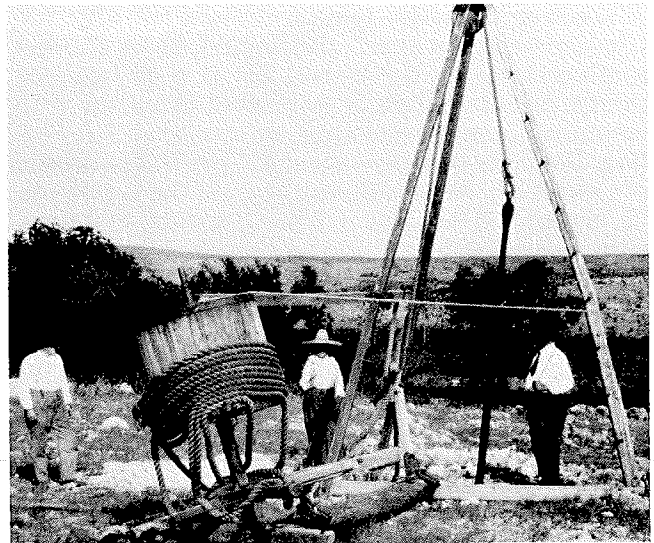
Figure 11. McGuire Mine, later named Ben Franklin Mine, SE-NE-SW sec. 21, T. 1 S., R. 1 E., Murray County, Oklahoma. View looking east, showing cable-tool rig that drilled test holes 125 feet deep. Results showed two thin ore beds in upper 30 feet and one bed 15–20 feet thick at depth of 125 feet. Dr. R. C. Hope on left, Gertrude Sober in middle, and C. Lincoln McGuire on right. Taken in Fall 1909. (Photo courtesy of Western History Collection, Bizzell Memorial Library, The University of Oklahoma.)
