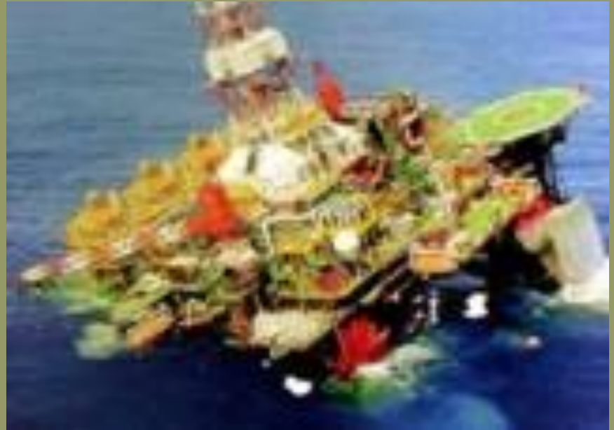
Semisubmersible rig sinking after being towed to site
