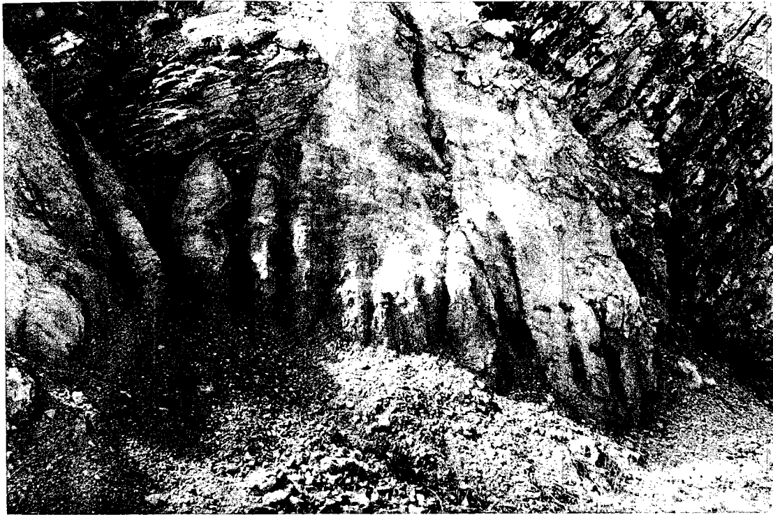
Figure 10. Collapse feature (sinkhole) filled with fine carbonate debris, mud, and large clasts. Note near-horizontal stratification that contrasts with apparent dip of host beds. Large ceiling block (above hammer) rotated into the cavern. I-35 road cut. Hammer for scale.
