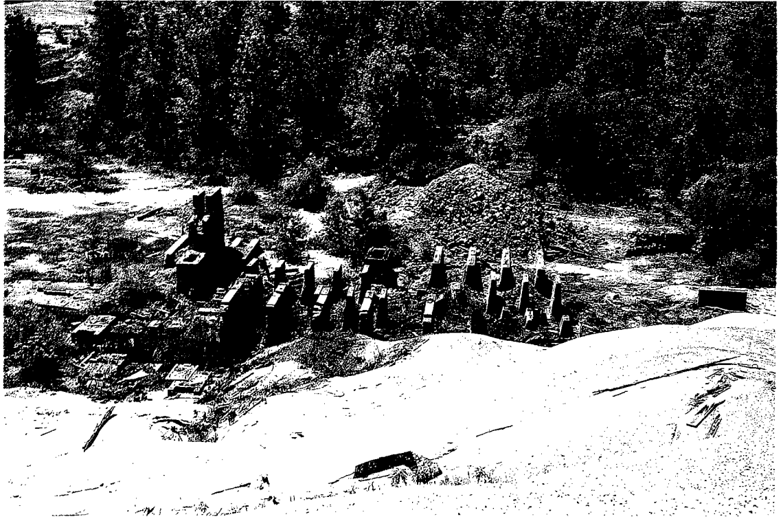
Figure 8. Foundation for former mill at St. Louis No. 4 Mine (29N-23E-24). Boulder pile is adjacent to mill, and chat pile is in foreground.
