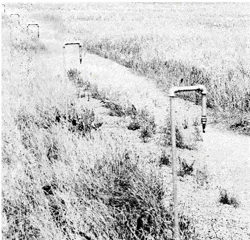
Series of fixed risers spraying effluent on small plot of Bermuda grass.
