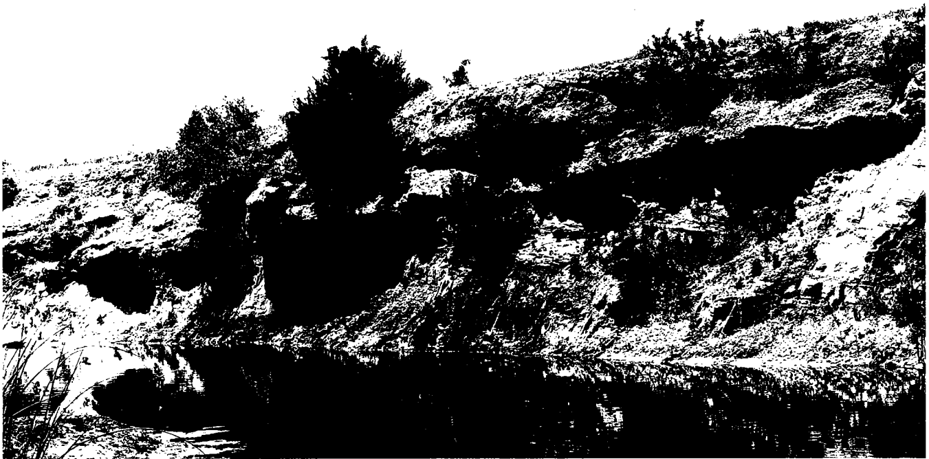
Figure 16. Two photographs of tar-sands quarry south of Sulphur. Above is view of open-pit mine that reached a depth of about 90 feet (27 m) before being abandoned in the 1950's. Below is a modern view of abandoned tar-sand quarry.
