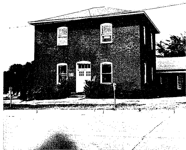
Figure 35. Supreme Court building of the Cherokee Nation, Tahlequah.
