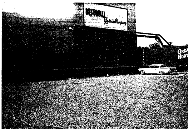
Figure 19. Bestwall Gypsum plasterboard and roofing dry-felt plant near Pryor.
